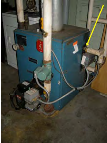
Typical older boiler (arrow indicates DHW heat exchanger)
