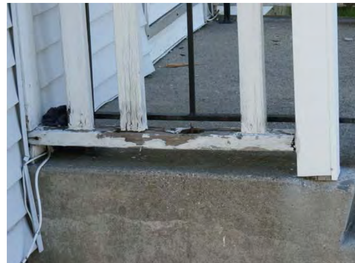
Example of porch deterioration
