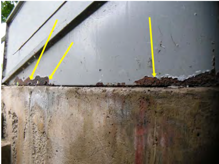
Typical bulkhead deterioration
