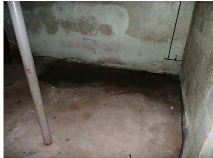
Typical example of basement water infiltration
