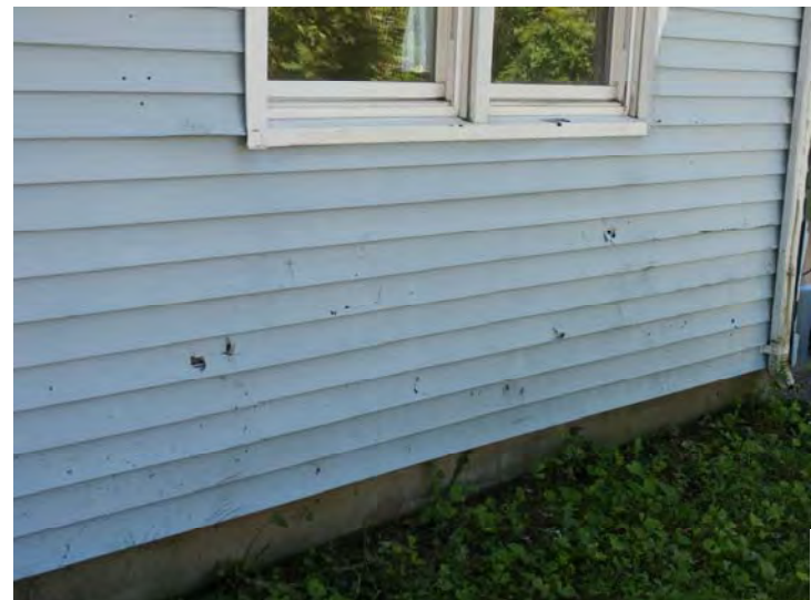
Example of common vinyl siding damage
