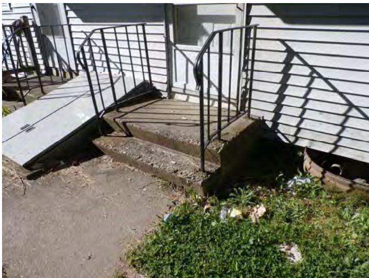
Typical example of concrete age related deterioration
